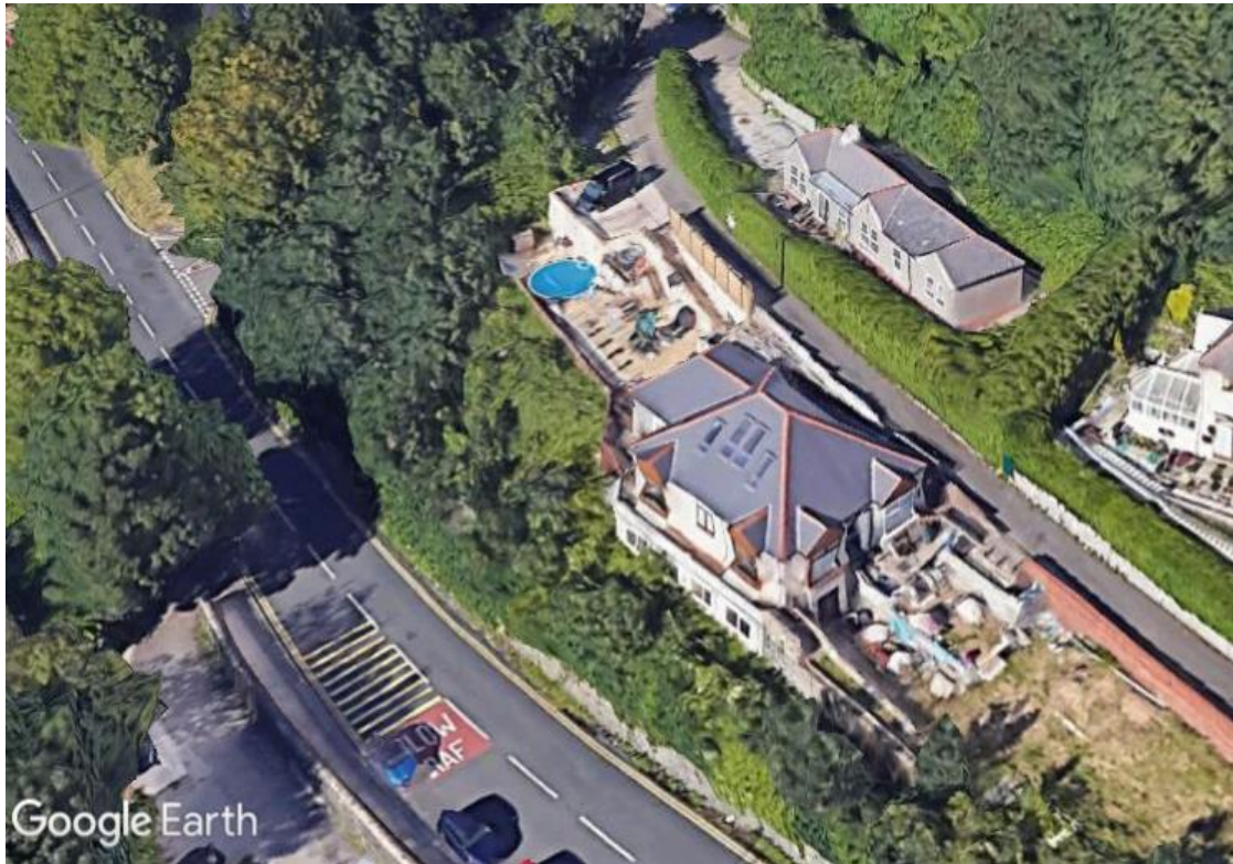
Figure 4 - Google Earth extract showing Number 26 in relation to the application site behind
